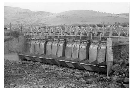
Discharge side of 650 CFS spillway located on the bank of a large canal that runs through a majorcity.
