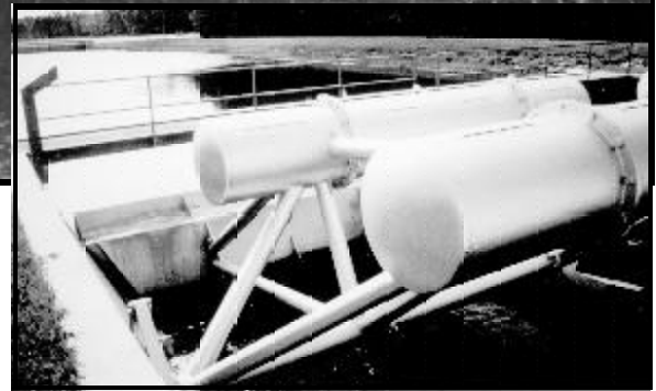
The Waterman Type C-21 gate, the largest in the series, is more than 26 ft. wide at the top. It is capable of regulating flows from almost zero to 2,000 cfs. Whatever the flow, the upstream level (seen here) will remain constant.
