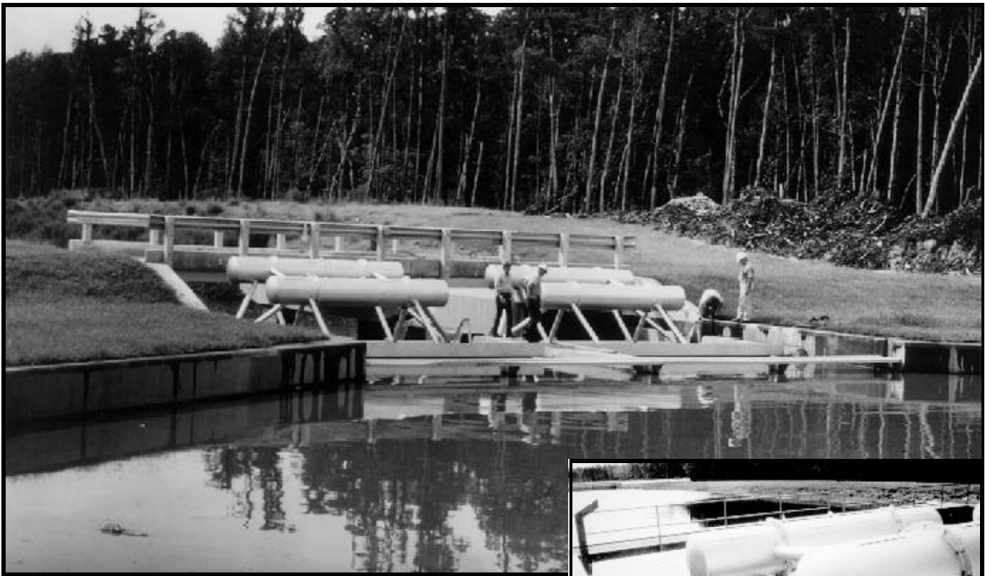
The Waterman Type C-21 gate, the largest in the series, is more than 26 ft. wide at the top. It is capable of regulating flows from almost zero to 2,000 cfs. Whatever the flow, the upstream level (seen here) will remain constant.
