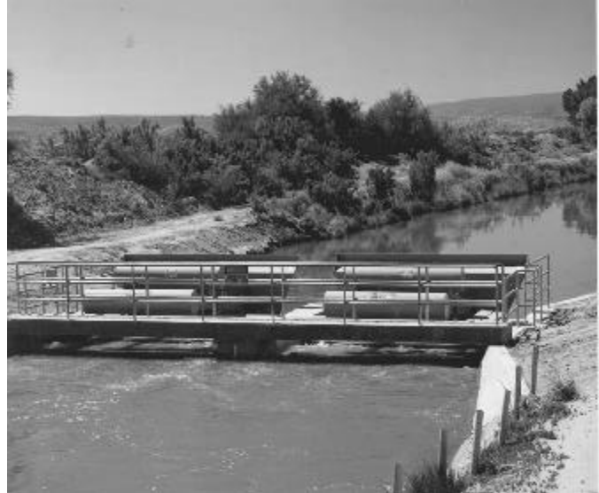
View from downstream.
